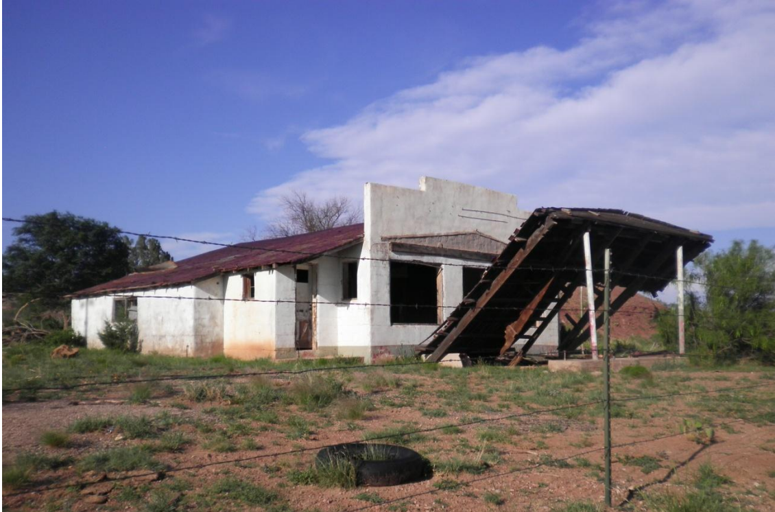
Plate 5. Unidentified building west of Endee New Mexico on Dirt 66.
