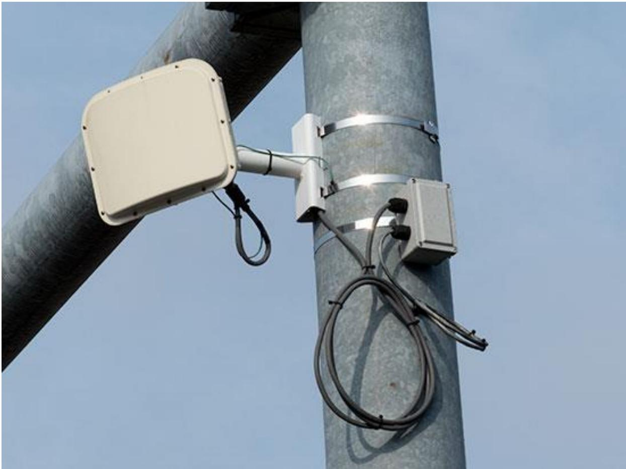
**Figure 2-2: Wavetronix Radar Detector (Huotari 2015)**
