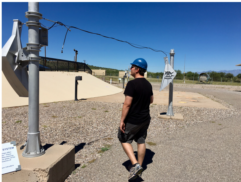
Figure 26. The author about to walk through a “tipsie”—these “scoops” created a radar beam between the two. When the radar beam was broken, it set off an alarm at the LCC.
