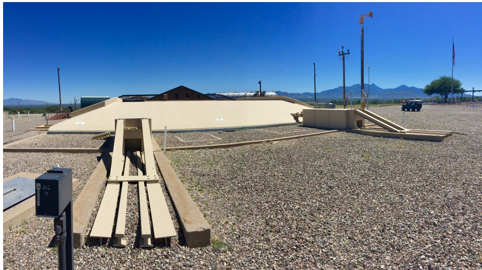
Figure 27. The missile silo door (topside) and skids that would direct the 750 ton steel and concrete door as it opened to allow for the missile to launch. Image credit: Taylor R. Genovese
