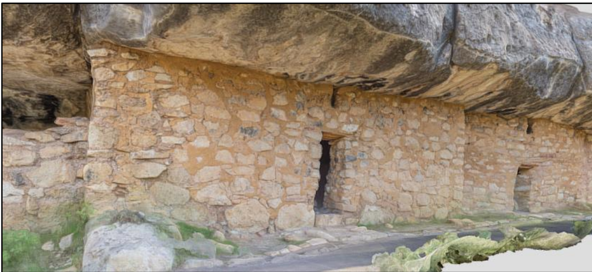
Figure 9. Model exterior view of Rooms A and B, facing northeast
